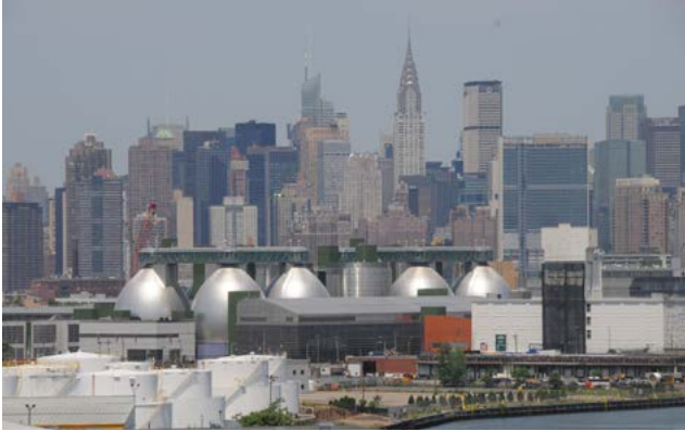
Anaerobic digestion facility at Newtown Creek WWTP Photo credit: NYC Department of Environmental Protection
